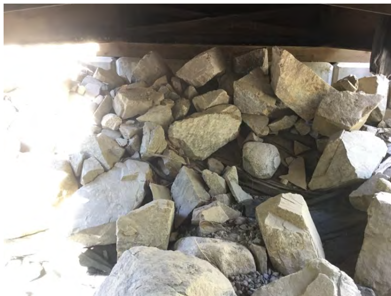
Right Bank Abutment when facing downstream
