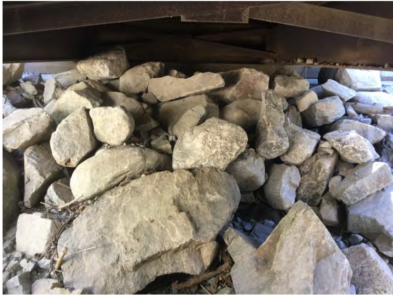
Left Bank Abutment when facing downstream
